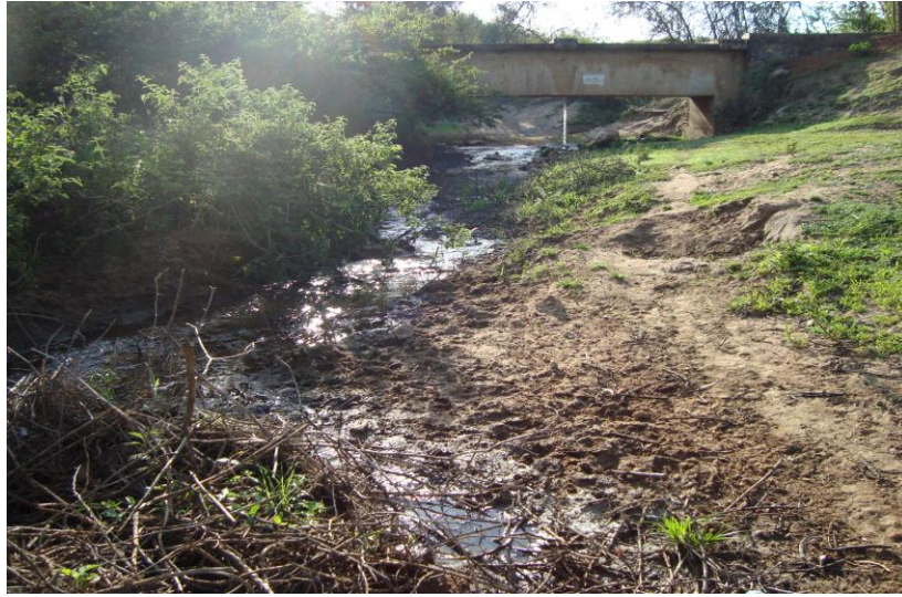
Plate 7.7. Water being conveyed through a sandy sub canal with the source from Yatta furrow feeding the downstream farms probably result to high seepage rates.
