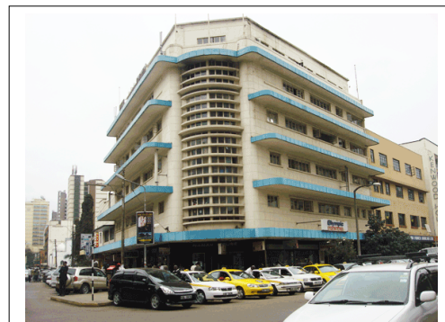
Plate 9.12: Scaling elements on Nanak House, by Author, 2010
