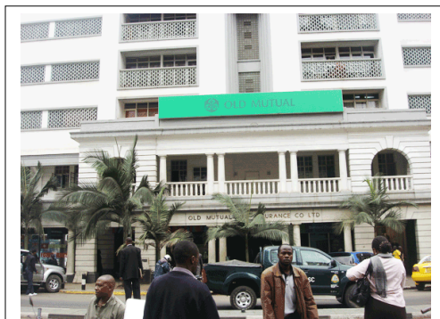
Plate 9.11: Colonnaded canopy on Old Mutual Building, by Author, 2010
