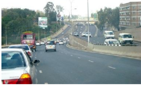
Plate 2.29: Wide Road in Nairobi, Kenya
