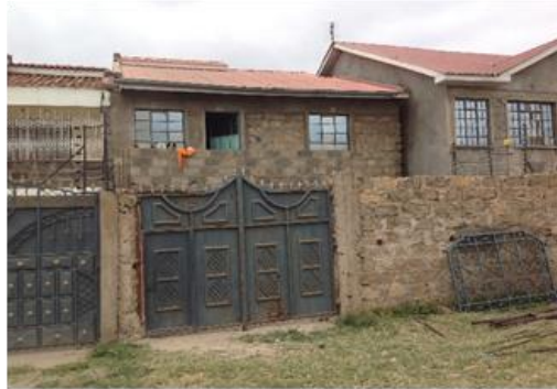
Figure 2.1: Occupied incomplete houses in Nasra Estate, Nairobi (source; Author, 2013)
