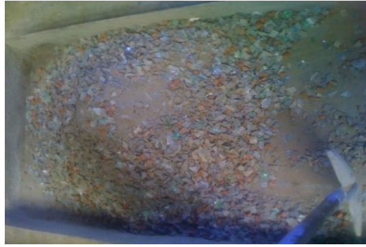
Plate 3.5: Manual concrete mixing using spade and tray
