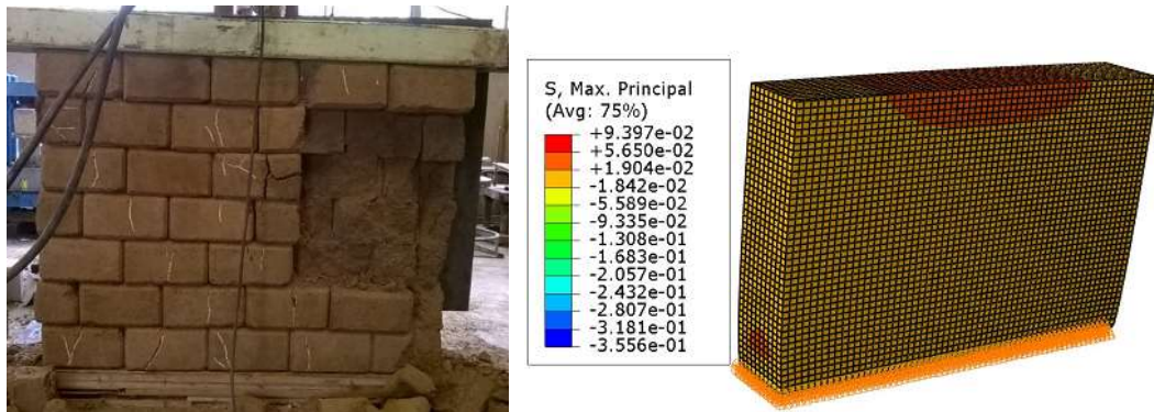
(a) Failure mode of experimental wall (LSW1) (b) Maximum principal stress distribution
