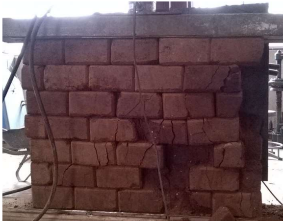
(a) CSW4 failure
