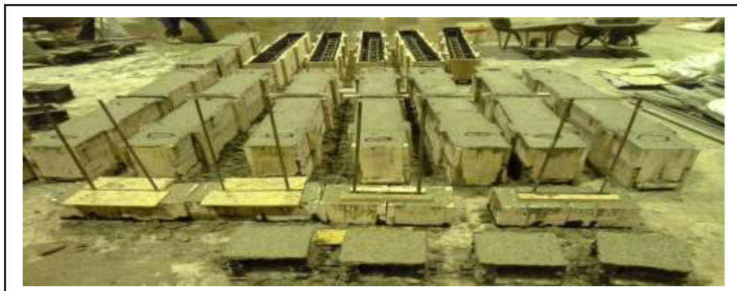
Plate 3.7: RC beam, concrete cubes and bonding cubes specimens after casting
