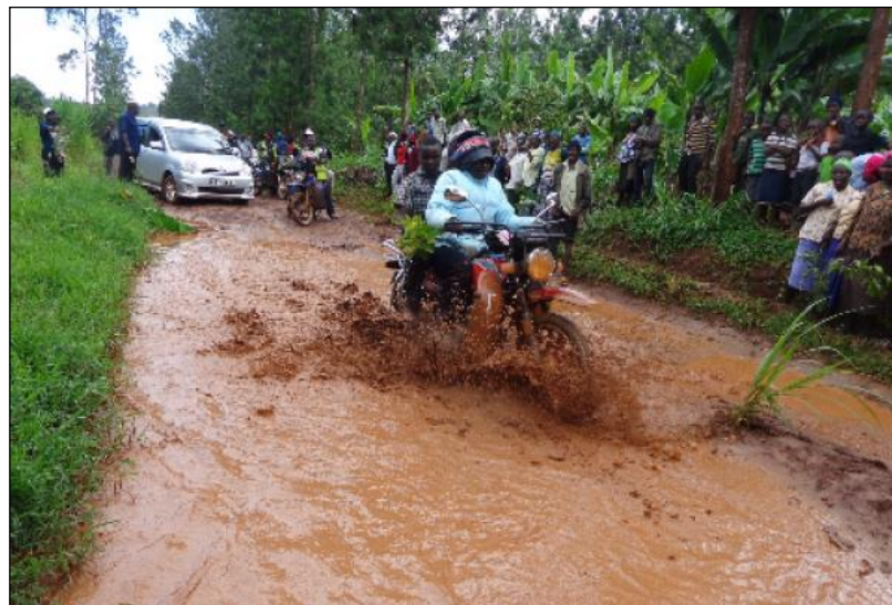
Plate 1.1: Bad condition of a rural road in Nyeri County during wet season
