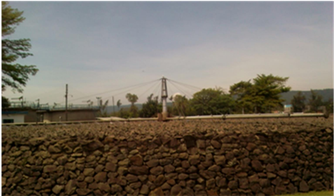
Plate 1.4: Trickling filter in Kisumu wastewater treatment plant (KIWASCO)
