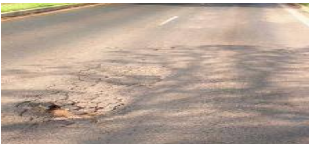
Figure 2.7: Pothole on wheel path area (Kamiti road)
