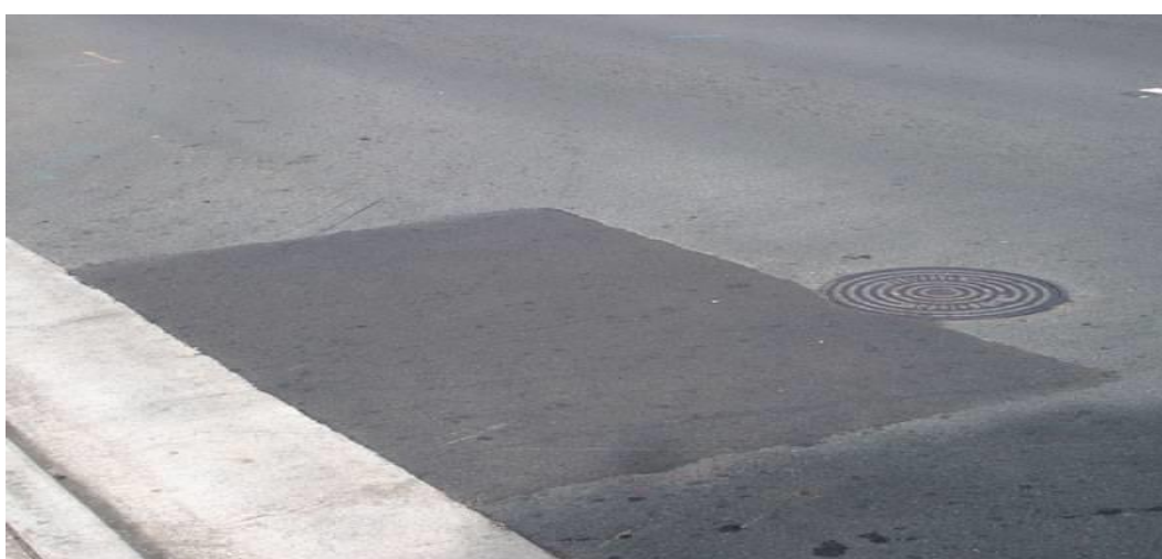
Figure 2.6: Utility patch on pavement (Kirinyaga road in Nairobi)
