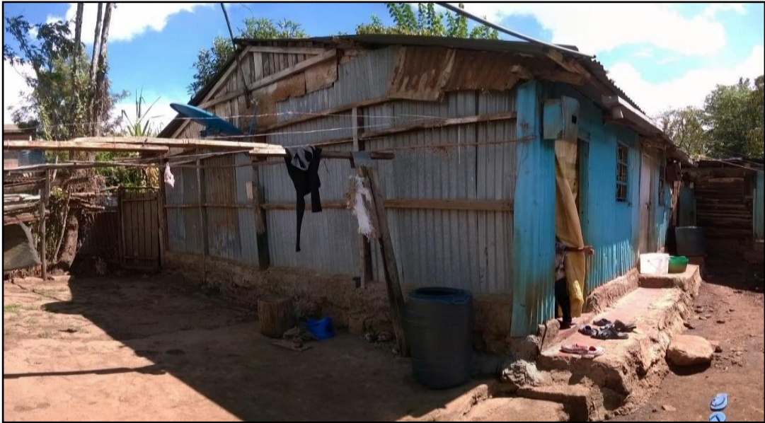
Plate 3.1: Two of the sheet metal clad buildings used in this study
