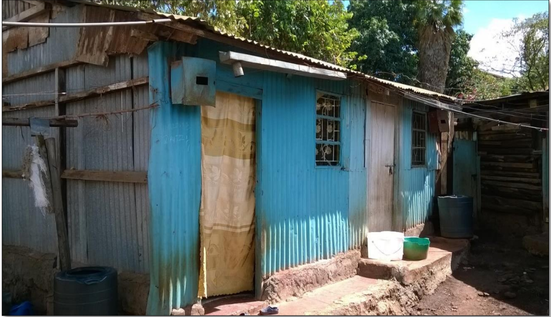
Vacant House A on the right side and occupied House B on the left (with curtain)
