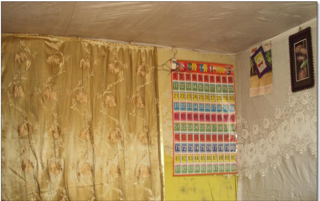
Data logger 3 was set on central partition wall in the sitting room area, House B
