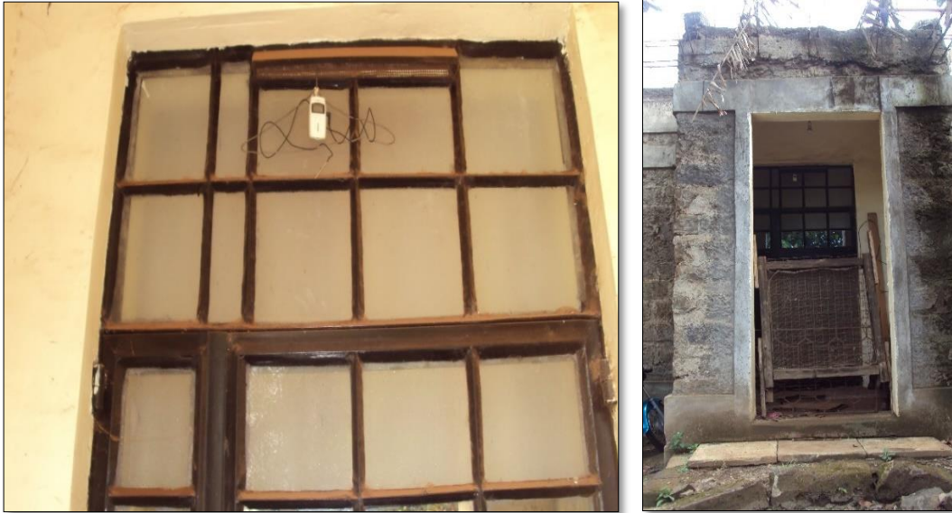
Data logger 1 located under canopy of stone and concrete building
