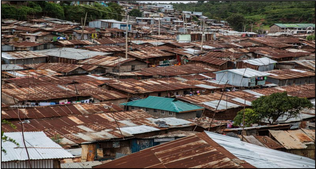
Plate 1.1: Sheet metal clad residential building settlement in Kibra, Kenya.
