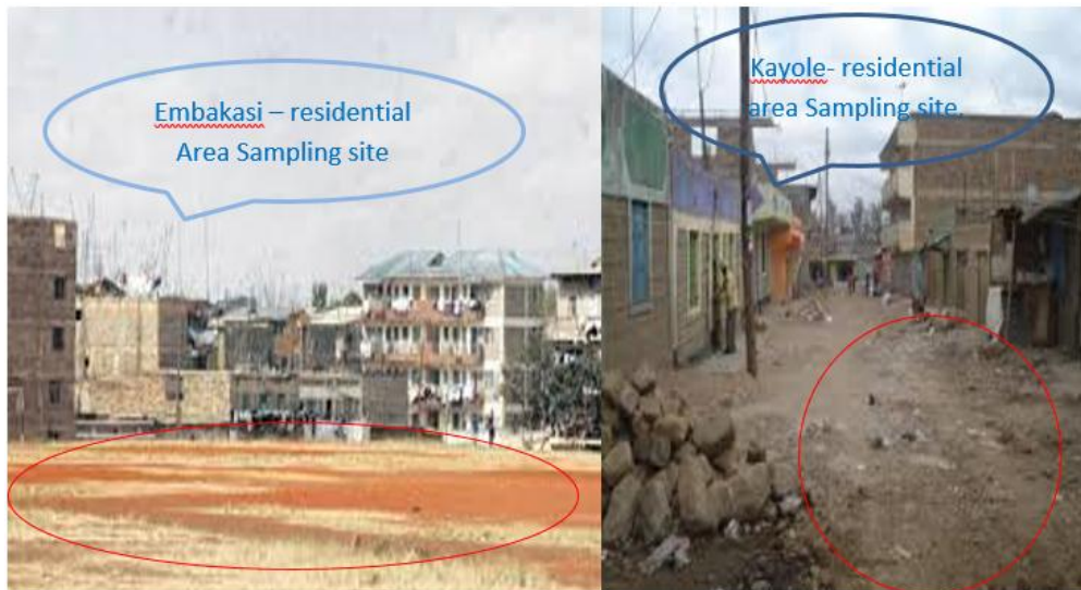
Figure 3:3: Dust prone emitting unpaved grounds and roads.
