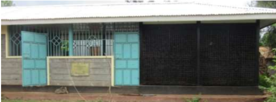
Figure 3.1: Evaporative charcoal cooler system with a preparation area.
