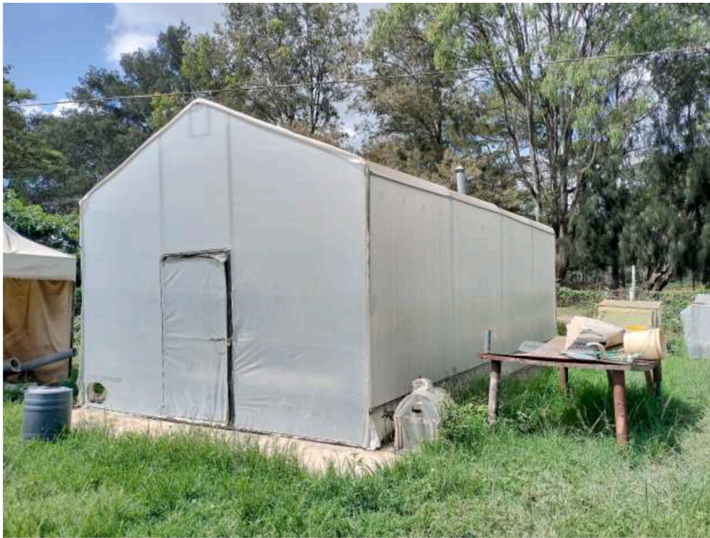
Fig. 1. Outside view of the solar-exhaust gas greenhouse dryer.
