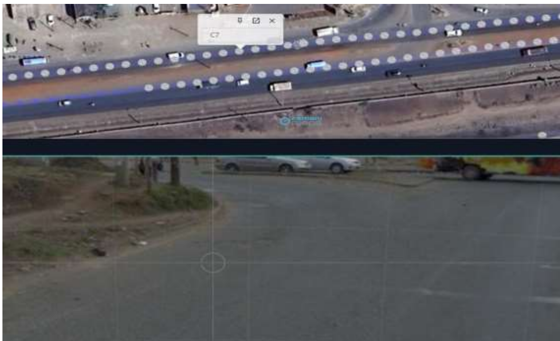
Figure 4.3: Road Surface Condition Highlighting Potholes along Mombasa Road
