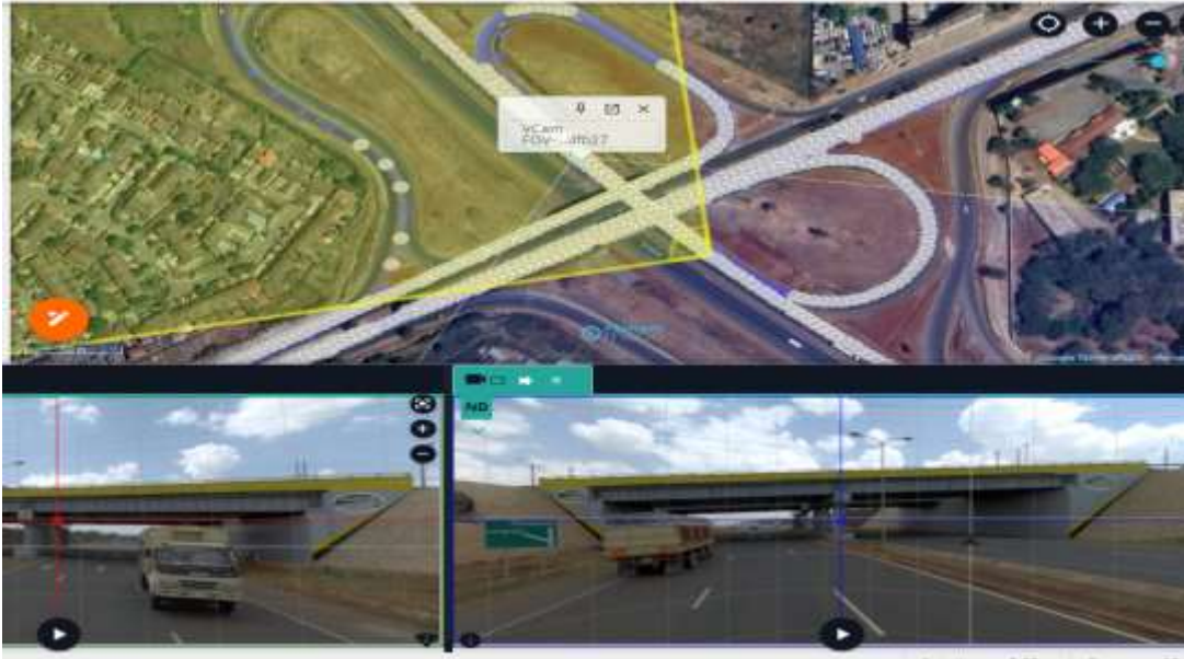
Figure 4.7: At Langata Interchange Showing Road Signage, Markings, Kerb and Streetlights
