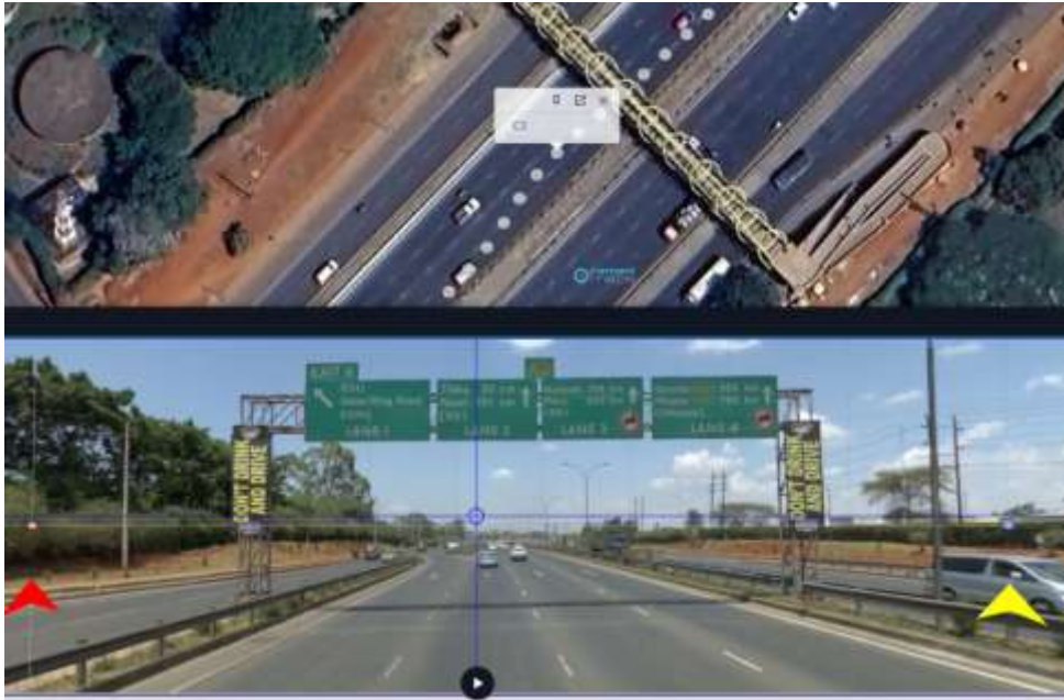
Figure 4.9: Thika Road showing the Road Markings, Signage, Guard Rails, Street Lights, Kerb
