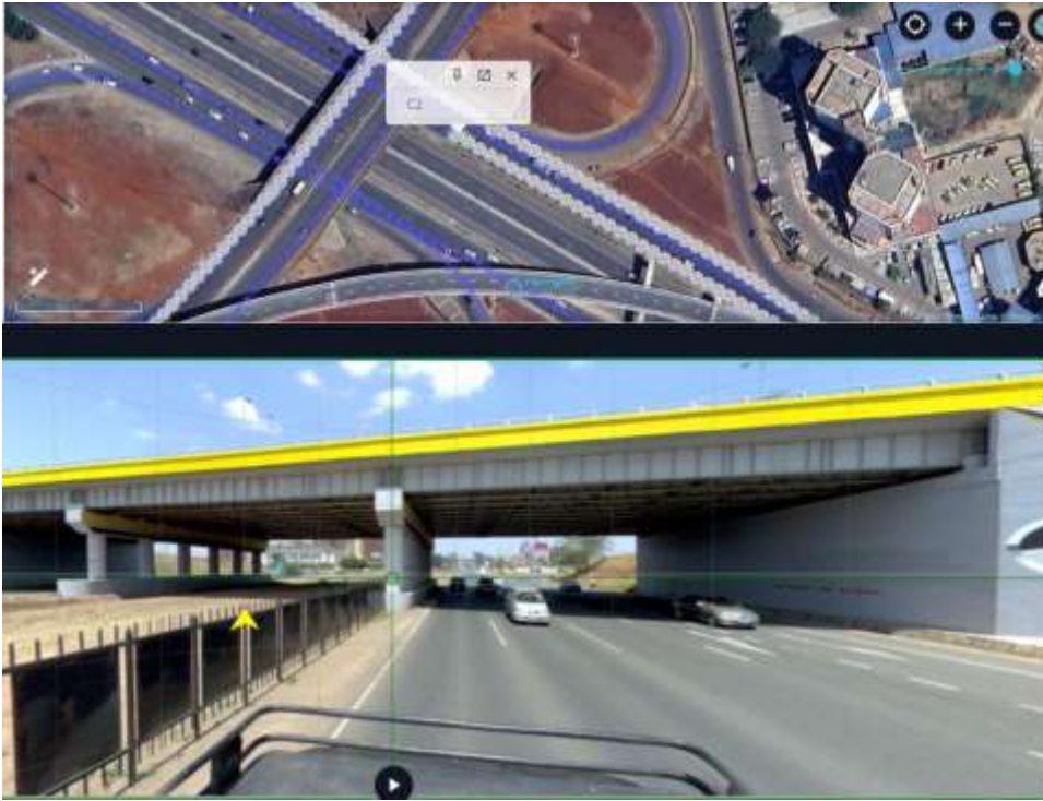
Figure 4.8: Mombasa road Interchange Showing the Road Markings, Kerb, Barrier as Well as Bridge Columns
