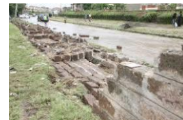
Fig 1: BRIDGE COLLAPSES DURING FLOODS
