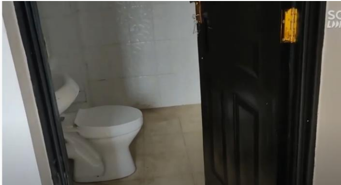
Figure 4.31:1-Bedroom Washroom (Source field survey)
