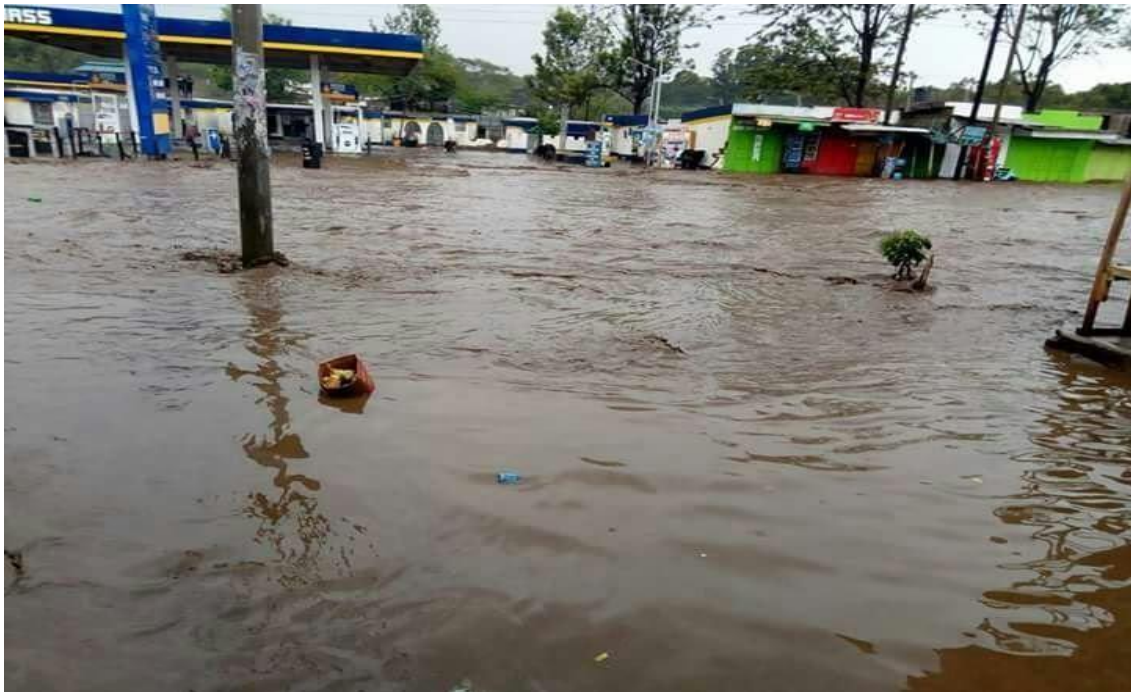
Plate 4.7: Built-Up Structures Submerged in Flood Water, Narok North Sub-County
