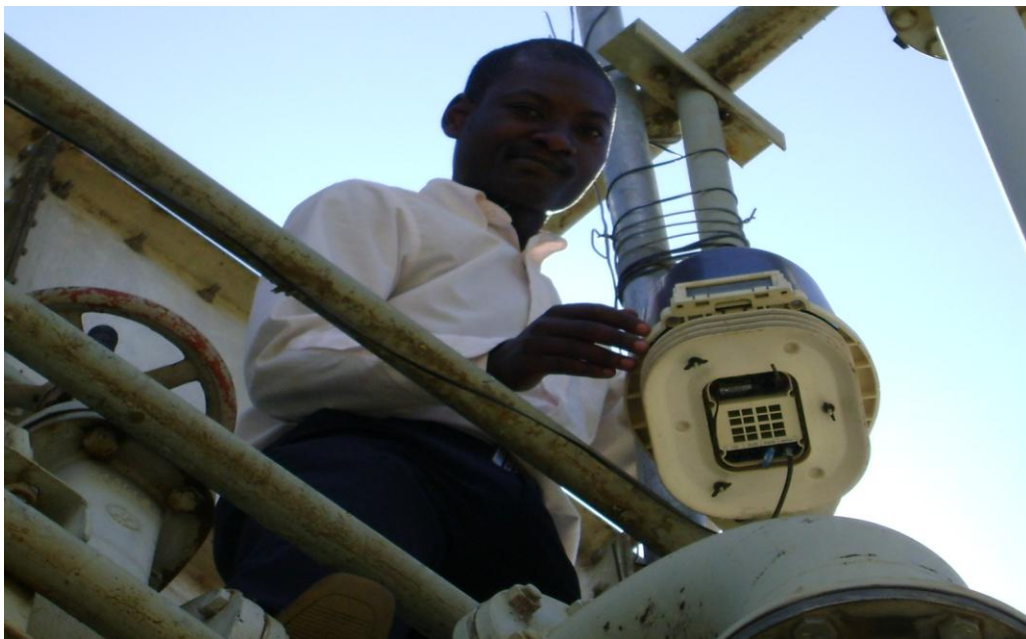
Plate 7: Clamping the transmitting device
