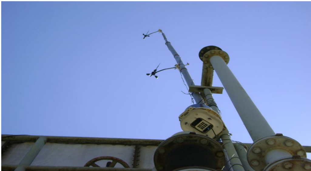
Plate 5: Mast clamped on to the supports
