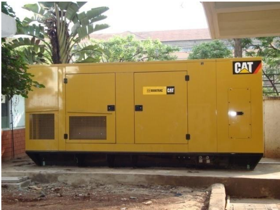
Plate 18 Recommended sound – proof housing for a power generator to reduce noise levels to acceptable values
